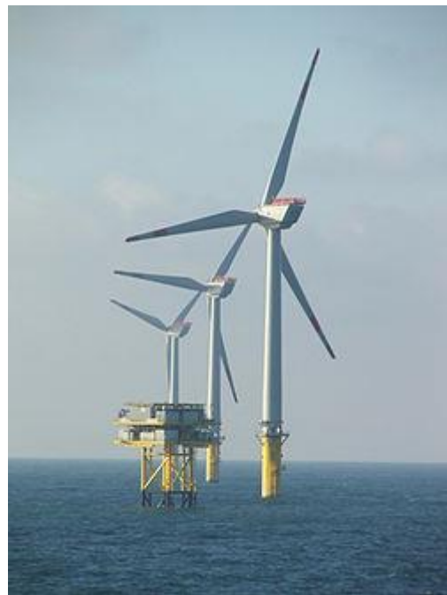
Fig. 2: - Wind turbines and electrical substation of Alpha Ventus supplied by Adwen in the North Sea
