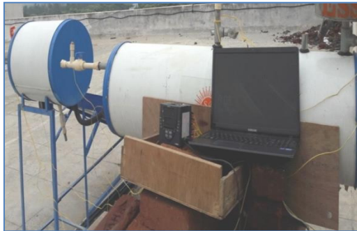
8 connections shown with data logger
