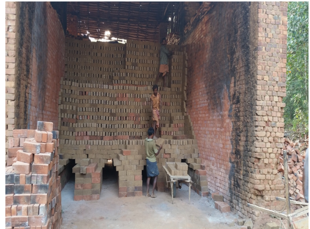
Fig. 6 Setting bricks in kiln
