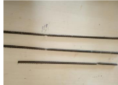
Fig 3(b) Failure of Deteriorated steel bars
