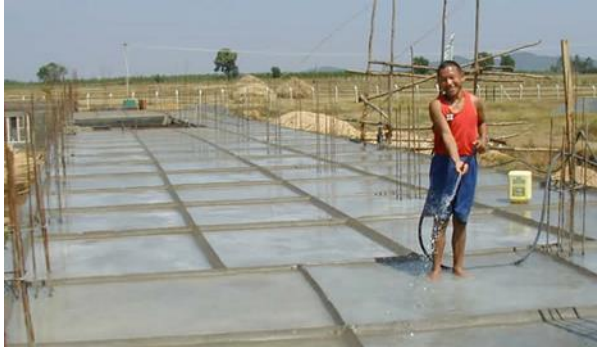
Fig. 2 Ponding method of curing
