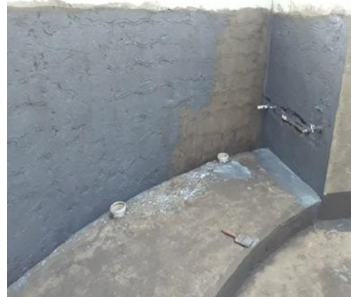
(a) During acrylic polymer-based waterproofing chemical coating (BeckProof WAC)
