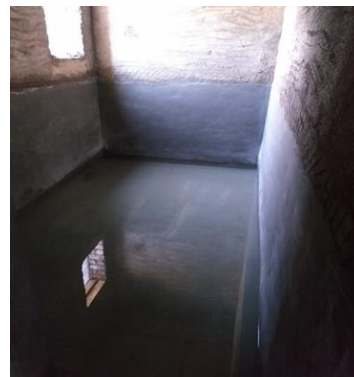
(c) After completing all above-mentioned waterproofing methodology procedure
