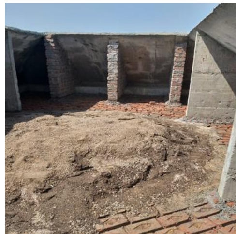
(b) During sunk filling procedure by using Brick bat coba system.
