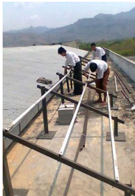
Fig. 7. Mounting the Structure Bar
