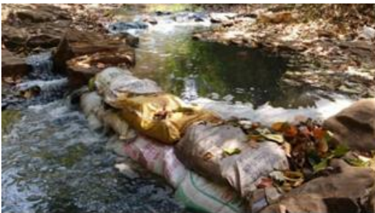
Fig No. 3. Construction of bund 2
