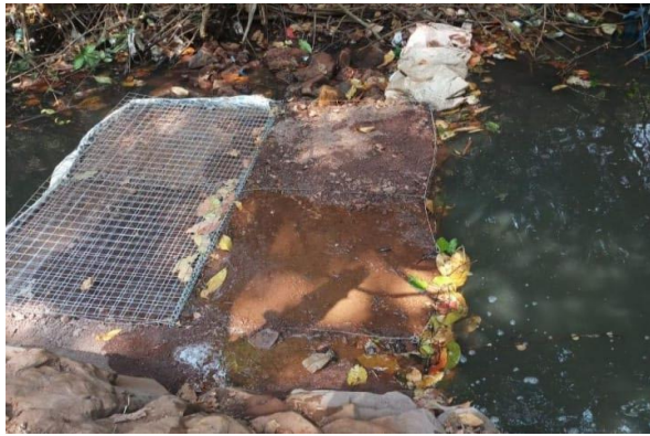
Fig. No. 7. Construction of Bed For plantati
