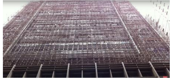
Figure 8 – Bamboo scaffoldings
