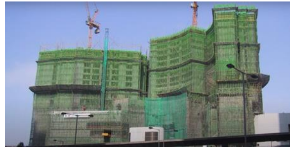
Figure 9 – Bamboo scaffoldings
