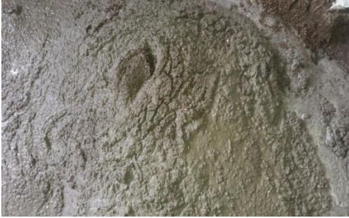
Fig.2 Wet Mixing of mortar with GBS
